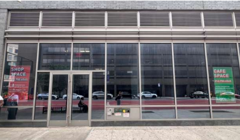
Retail 4 Frontage on Livingston Street
